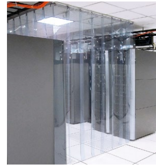
Overlapping Strip Curtain Doors Overlapping vertical strips provide effective and efficient approach to sealing aisle entry way.
